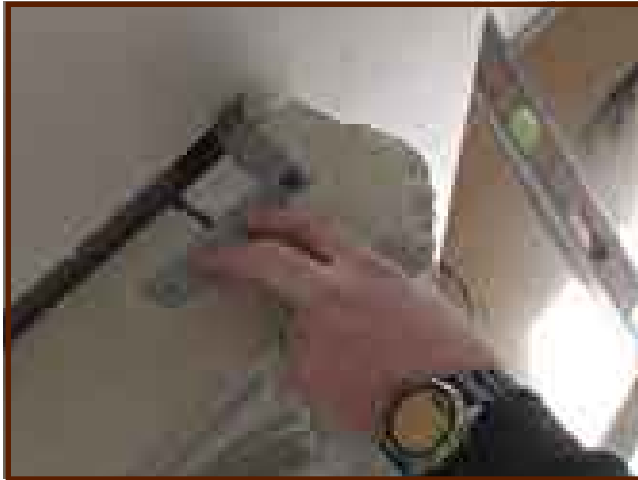
Above, the mason drills a pilot hole to anchor leg to wall.
