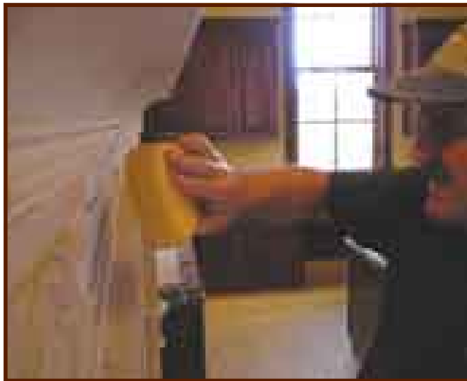
Above, the mason drills a pilot hole to anchor leg to wall.
