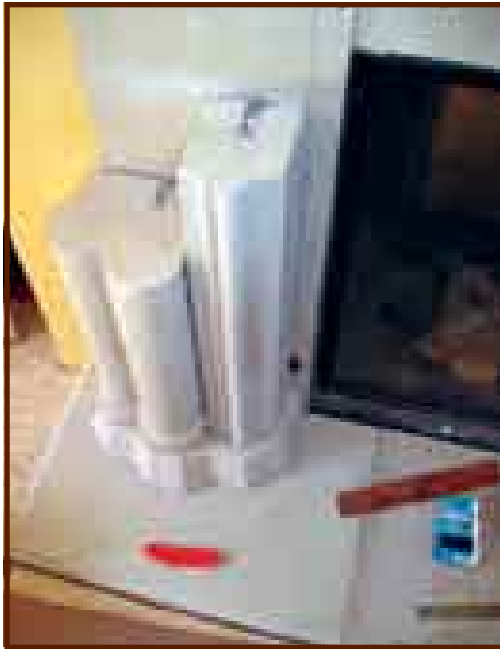
Once the hearth is set, the legs are carefully put into place and tied back to the framing. Note the ties in the tops of the stones in the photo above left. At right, the mason is checking joint spacing on the next layer.
