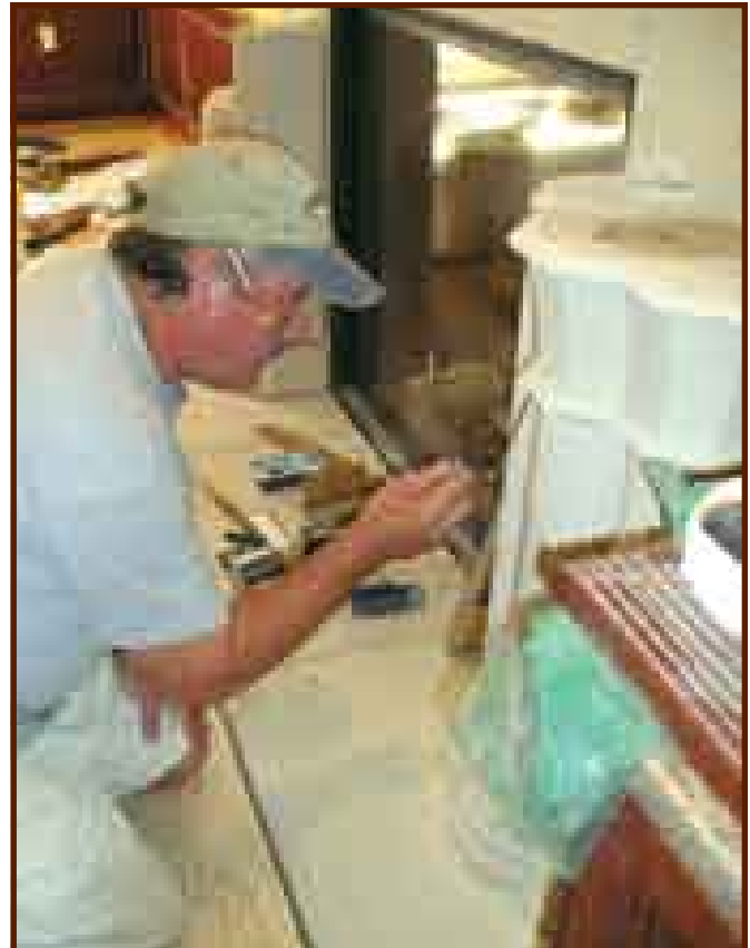
Once the hearth is set, the legs are carefully put into place and tied back to the framing. Note the ties in the tops of the stones in the photo above left. At right, the mason is checking joint spacing on the next layer.
